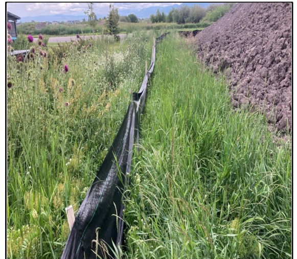
Fig. 1: Compliant residential job site
