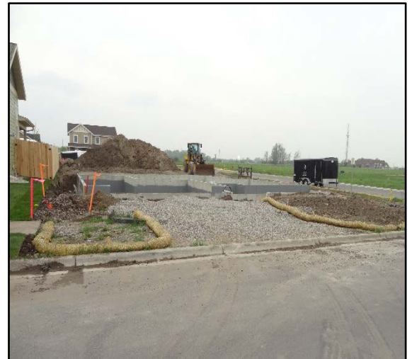
Fig. 1: Compliant residential job site
