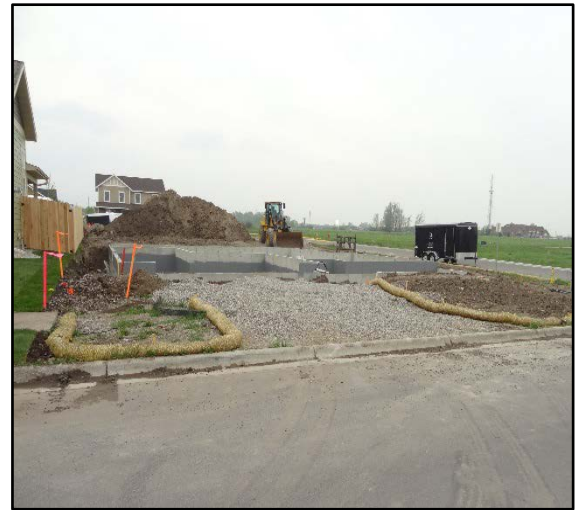
Fig. 1: Compliant residential job site
